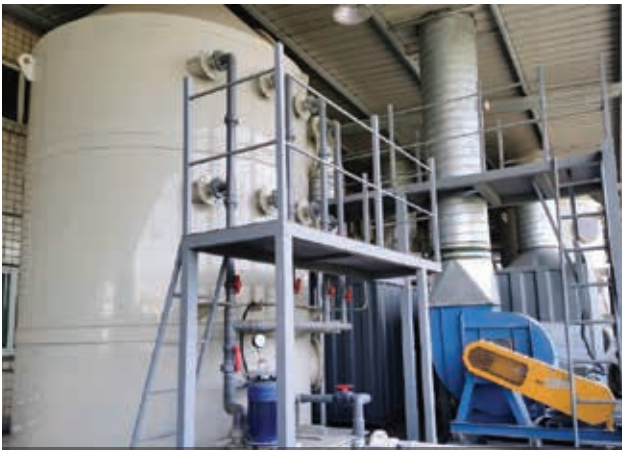
Fu Yu Suzhou – Exhaust Gas Treatment System for Moulding Department
