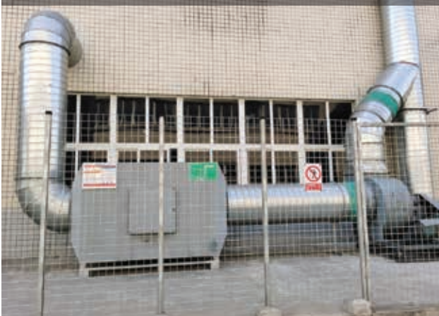
Fu Yu Suzhou – Exhaust Gas Treatment System for Moulding Department
