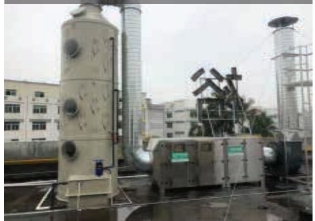
Fu Yu Dongguan – Exhaust Gas Treatment System for Moulding Department
